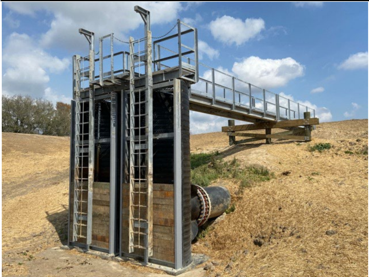
Figure 25: Double weir in the Savannah District, showing ladders, weir boards, and tie-point attachments for a safety lanyard to be used while ascending and descending the ladder. Fall protection should always be worn when working around a weir.
