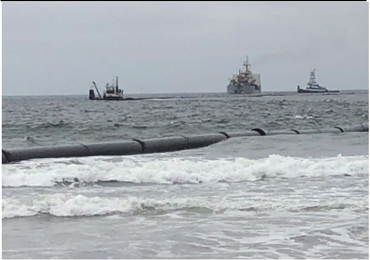
Figure 18: Pipeline connecting to the Dredge Stuyvesant for pump-ashore (pump-out) beach nourishment work. The tender and tug vessels are used to maintain the anchors on the pipeline.
