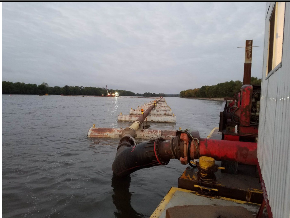
Figure 22: Inland river dredging discharge barge (looking upstream toward the dredge). The floating pipeline has several amber lights for visibility (required for safety). Associated navigation notices (notice to mariners) are broadcast that request mariners to radio the dredge at least 30 minutes prior to transiting the area. Each contract will specify the person responsible (usually the contractor's CQC) for distributing the notice to mariners. The QAR should confirm that the notice is distributed and accurately describes the work area. (Photo from Rock Island District)
