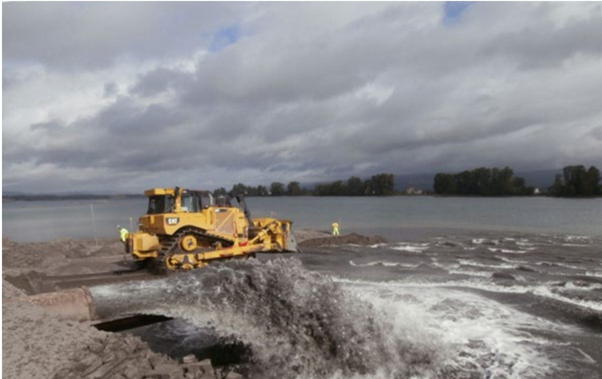
Figure 17: Discharge of a pipeline. Discharge can be directly into an enclosed site, into the open water, or onto a beach. Discharged material is moving at a high velocity and can cause injury. The area of discharge should be avoided because pumping can begin at any time. (Photo from Portland District)
