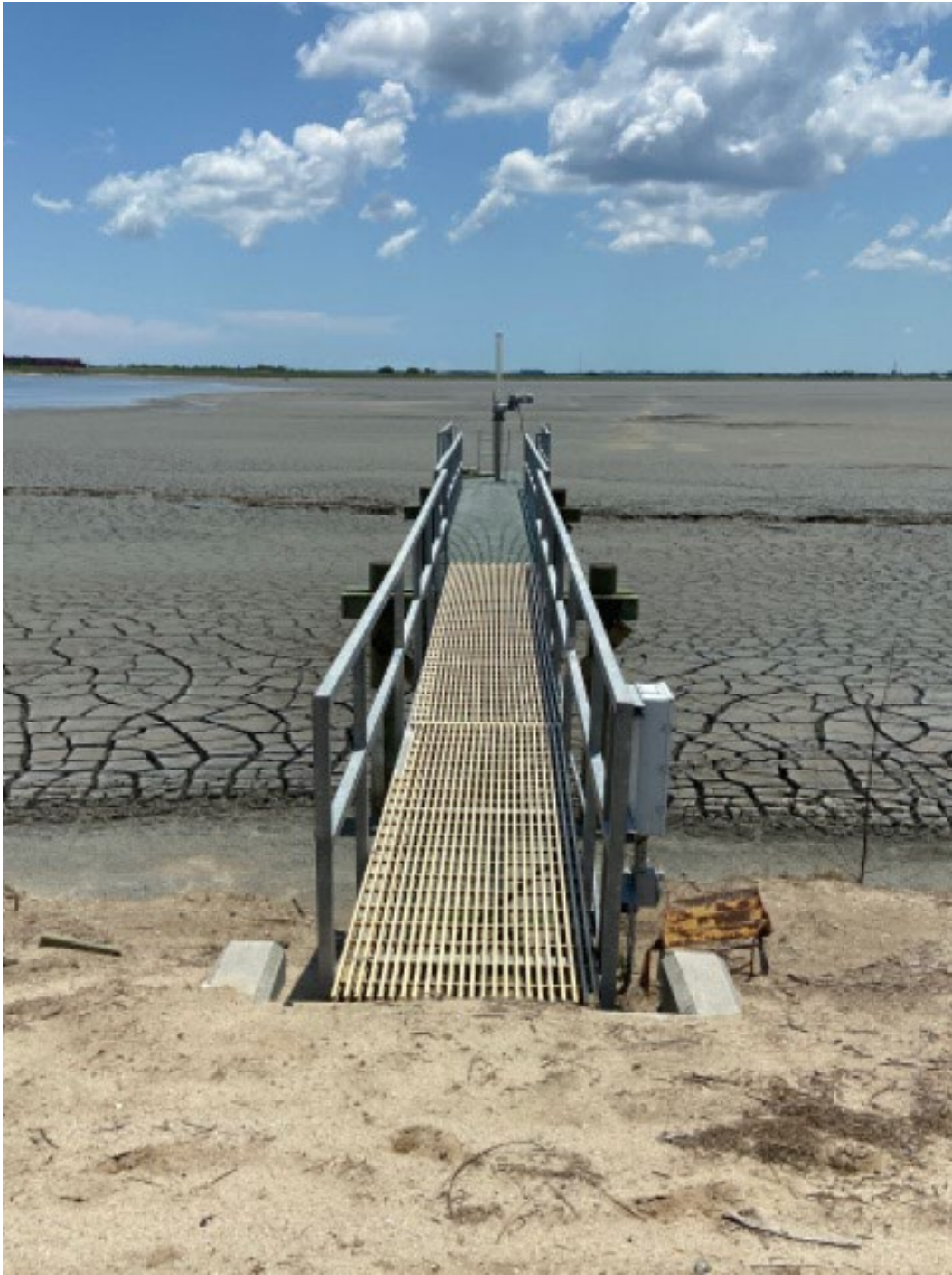
Figure 26: Catwalk to a weir structure. Placement area shows crackled “false surface” that forms after water has been partially decanted but can give way when stepped on. Always use the catwalk when accessing a weir structure but inspect it for structural soundness prior to use (check for signs of deterioration, such as rust, which could result in failure).
