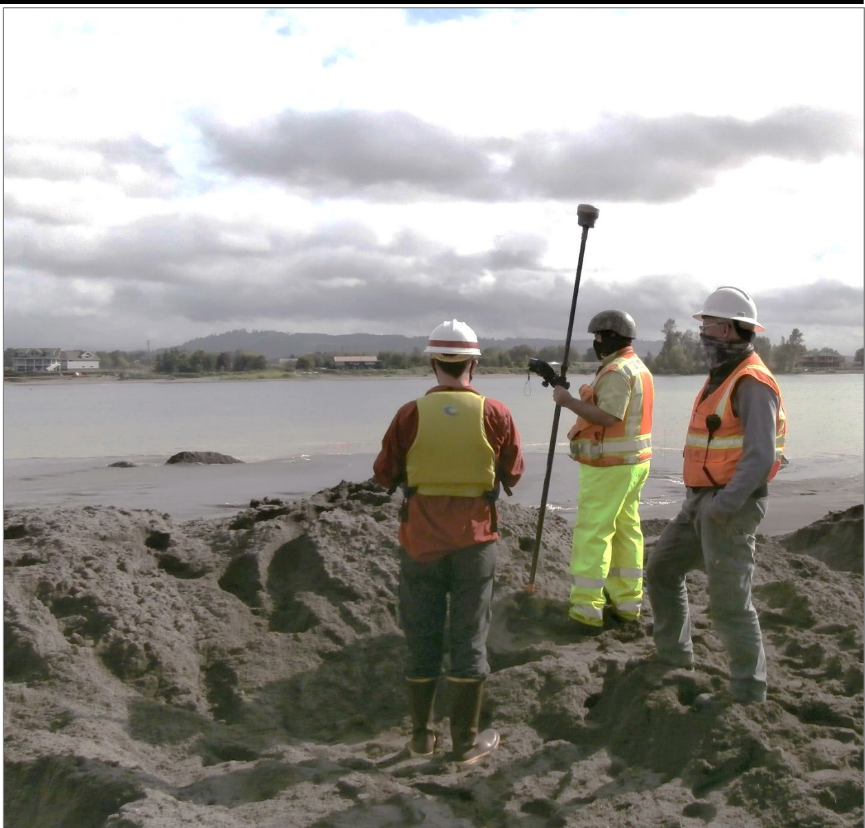
Figure 29: The personal protective equipment (PPE) worn at the placement site in this photo includes hard hats, high-visibility safety vests, personal flotation devices, shirts with sleeves, long pants, and closed-toe boots. Eye protection and hearing protection are other commonly required PPE.
