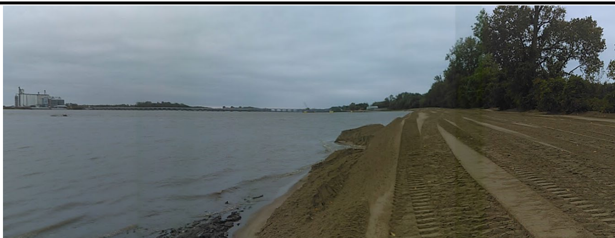
Figure 21: Example of site after hydraulic bank line placement followed with post-placement grooming by bulldozers used to knock down the high spots, a common practice along the Mississippi River (Photo from Rock Island District)
