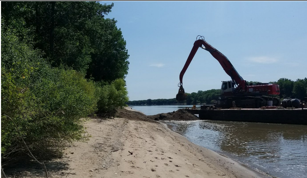
Figure 20: Example of mechanical dredge performing bank line mechanical placement on an inland waterway. Considerations for this type of placement are to reduce the encroachment of the material into the waterway by getting as close to the bank line as possible. In some cases, a backhoe may be stationed on the bank to pull material onto the shoreline and then push the material up to the natural tree line. Covering the exposed roots of mature trees with the material is done to prevent established trees from falling into the river and degrading the bank line. Material tends to stay on the bank longer if it is placed closer to the natural tree line. Sites may need to be surveyed for species of concern before placement. (Photo from Rock Island District)
