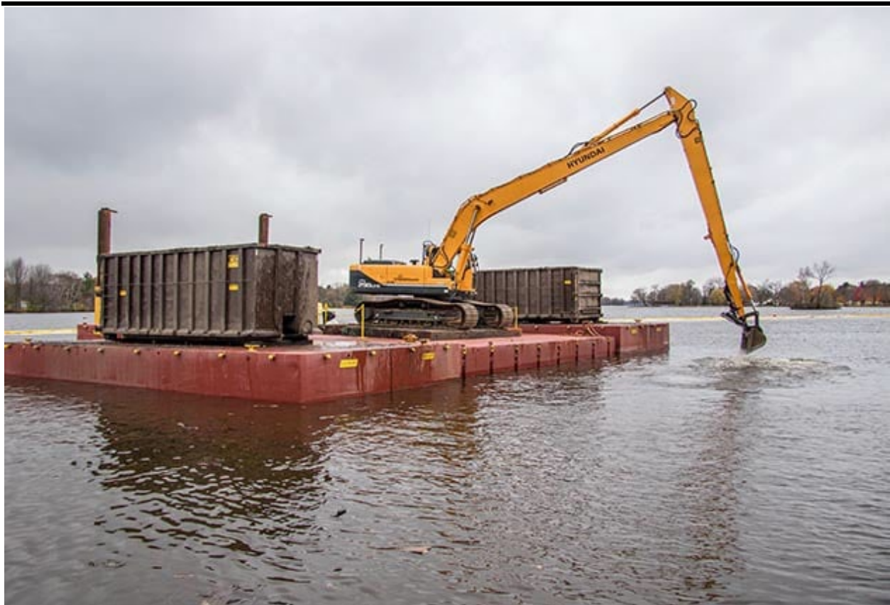
Figure 15: Excavator (mechanical) dredge on barge. Excavator dredges are limited in their dredging depth capabilities but can be precisely controlled so there is less danger when dredging around structures. (Photo from J.F. Brennan)
