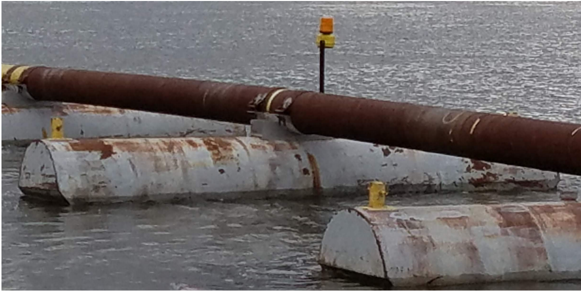
Figure 23: Detail of an amber light marking a floating pipeline on an active dredging job (Photo from Rock Island District)
