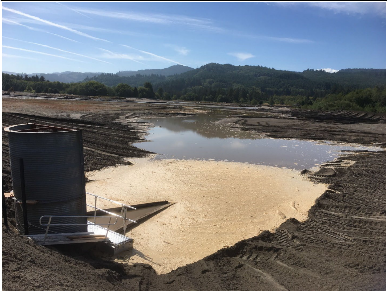
Figure 28: Upland placement site in Portland District. The catwalk and handrail are on floats and adjust to the fill level of the site. Weirs are removed after the site fills up or after placement is complete. The catwalk provides access to the front of the weir to adjust weir boards. Fall protection and personal flotation devices (PFDs) are required because of gaps in the handrails.
