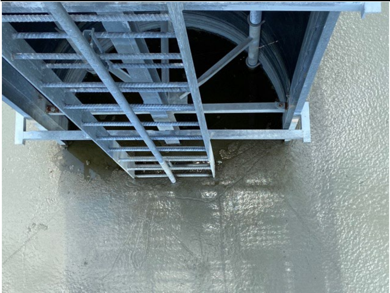
Figure 27: Looking down from the top of a weir ladder in the Savannah District. Muck and mud have accumulated around the weir boards and submerged the bottom of the ladder. Ladders that been submerged for extended period of time can decay and should be inspected for soundness before use.
