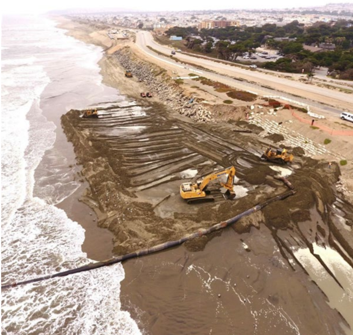
Figure 19: Beach placement using pump-out from a hopper dredge in San Francisco District. Note the orange safety fencing in the background to keep the public away from the workspace. Security guards were employed onsite. In this location, the sand berm over the pipeline was used to maintain emergency services access.
